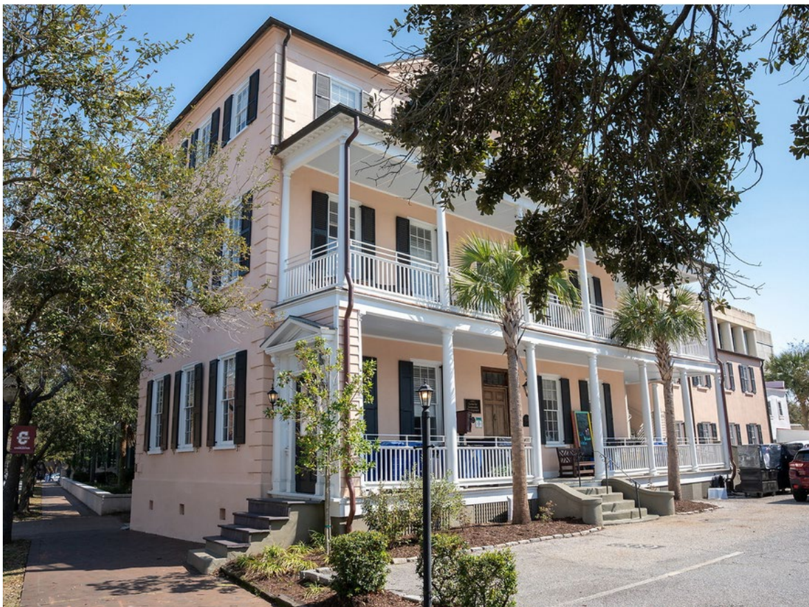
207 Calhoun Street exterior construction is complete
