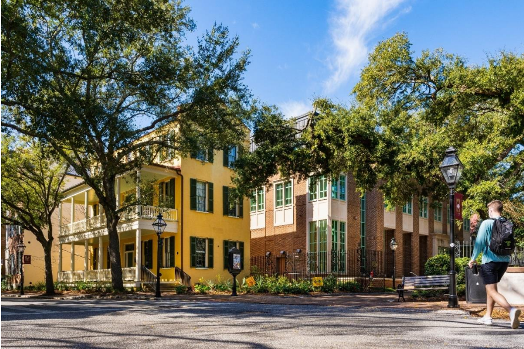
Historic buildings nestle beside the state-of-the-art Rita Hollings Science Center at the corner of College Way and George Street.
